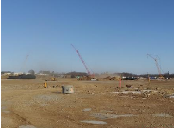
Middle of the site looking North (01/27/2022)
