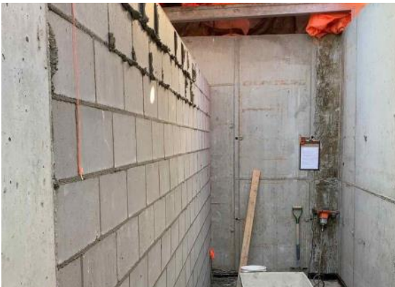
Lower level of elevator shaft in the auditorium (01/25/2022)
