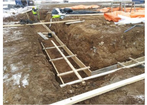
Concrete footing forms in future lab space (01/13/2022)
