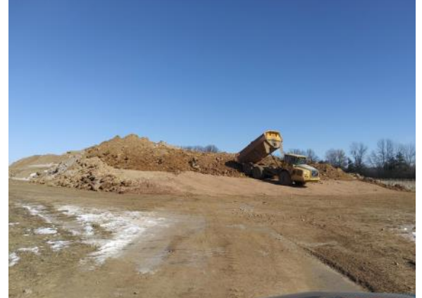
Spoil pile in south part of the site (01/27/2022)
