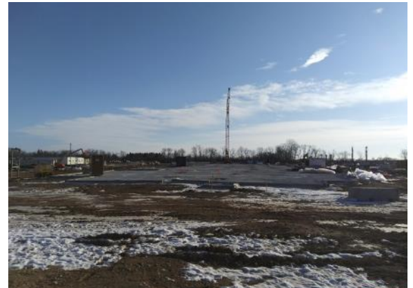
Looking East at all four classroom wings (01/27/2022)
